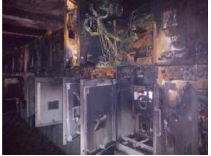
Falling of Kikar tree on 11 KV Behrampur & 11 KV UPS-1 feeders on dated 1.1.2016 lead to heavy fault & switches of both the feeders as well as 11 KV Breakers got burnt
