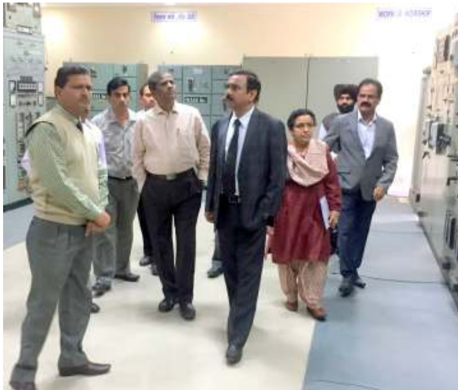
220 KV Sub-Station Ablowal (Patiala) Control room
