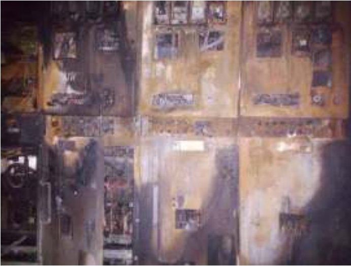
Falling of Kikar tree on 11 KV Behrampur & 11 KV UPS-1 feeders on dated 1.1.2016 lead to heavy fault & switches of both the feeders as well as 11 KV Breakers got burnt
